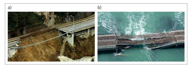
**Figure 1** Examples of Recent Transport Infrastructure Failures a) Landslide in Switzerland, 2005; b) Viaduct collapse, Ireland, 2009
