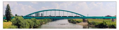
Figure 3 Static testing of the bridge "Sava" - two compositions in the main span
