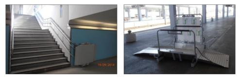
Figure 8 Ramp for the disabled persons in the pedestrian underpass of the railway station Vinkovci and elevation platform
