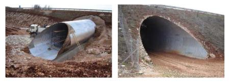
Figure 9 Installation of animal underpass – phase II and animal underpass in km 5+030,00 of Adriatic Highway – ISTRIAN "Y"
