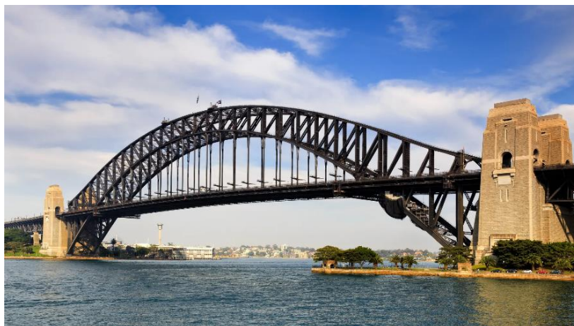
Slika 3. Sydney Harbour Bridge ( https://encrypted-tbn1.gstatic.com/images?q=tbn:ANd9GcTbtyzbZbH_THW0kX24iozHwsl1yl2YjVV0gnLnWtbaQcJBdel )
