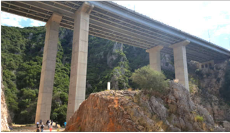
Figure 2 Egnatia Motorway G4 Bridge (© EOAE)
